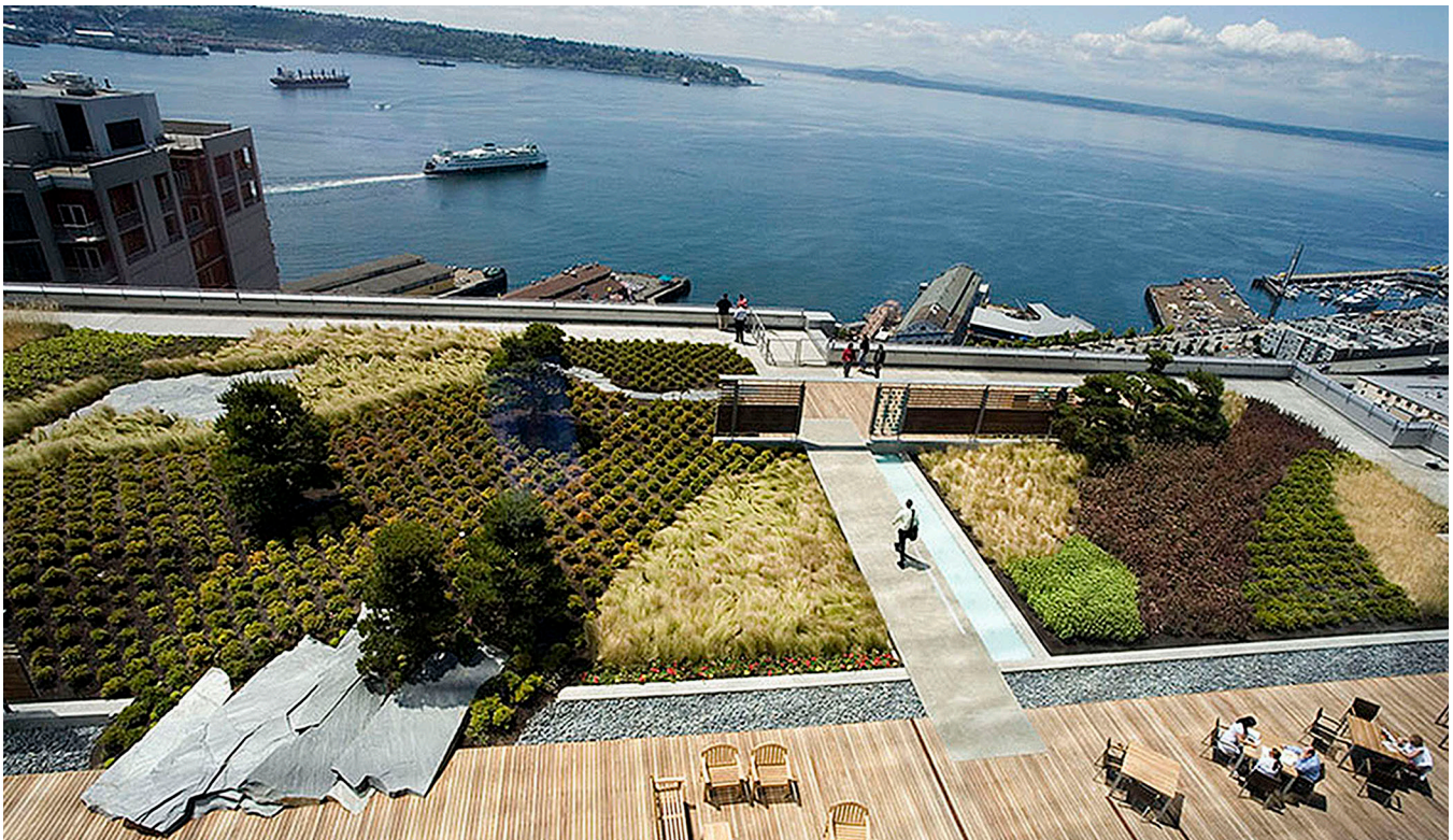
Pictured: The Russell Investments Center (formerly owned by Washington Mutual Bank) is one of the largest green roof installations in Seattle. Offering sweeping views of the Olympic Mountains, Mount Rainier, and Elliott Bay, the 17th floor green roof features predominantly native, drought-resistant planting and transformed a previously windowless lunchroom into one of the best tenant spaces in the City and helps manage their stormwater runoff.
