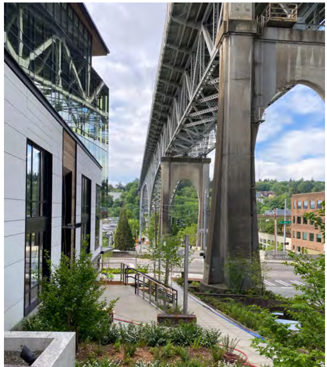
Pictured: The Watershed project by District members Weber Thompson and Stephen C. Grey & Associates which went through the Living Building Pilot program and will harvest and recycle 150,000 gallons rainwater annually. In addition, the project treats 300,000 gallons of runoff from the Aurora Bridge and connects to the Data 1 swales on the adjacent site.
